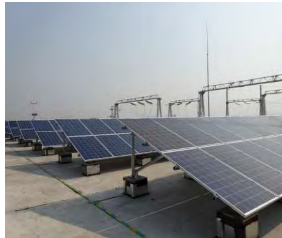
Project Location: Shanghai, China Capacity: 60MWp Completion Year: 2018 Type: Ground Mounted
